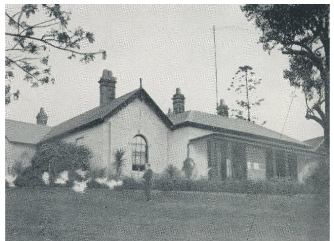
THE CLUBHOUSE IN 1912 showing the wireless mast
